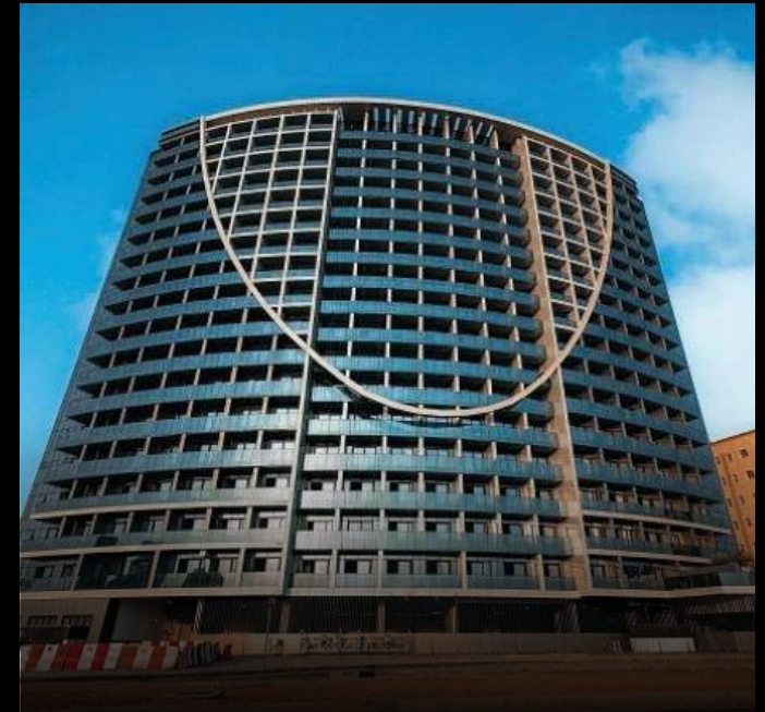
The V Tower Dubai Land
