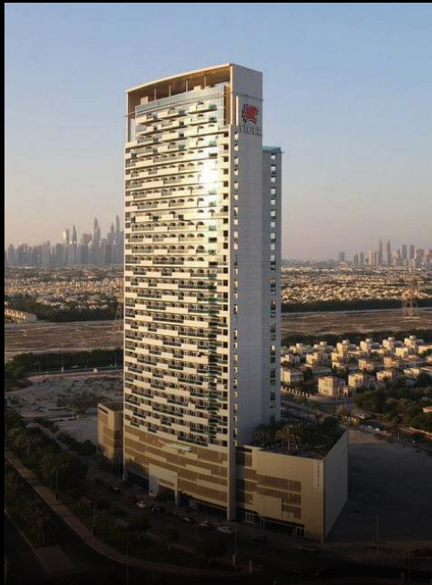
Al Jawahara Tower JVT, Dubai
