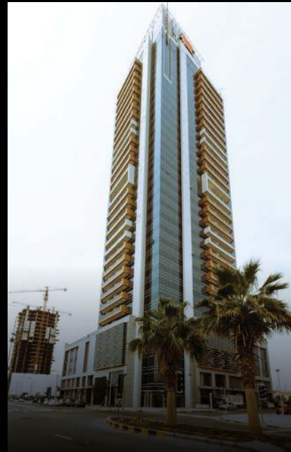
Al Manarah Tower JVT Dubai
